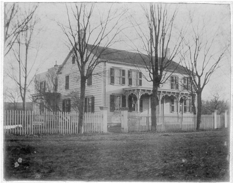
Figure 3. View of the Wehnau house, looking southeast, c.1898. The Italianate porches have been added, as has the flat roofed two-story wing at the northeastern corner of the building. Similar porches were added to the Philips house on Philips Road in East Greenbush, c.1878.
